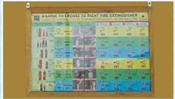
Information on Fire Extinguishers
